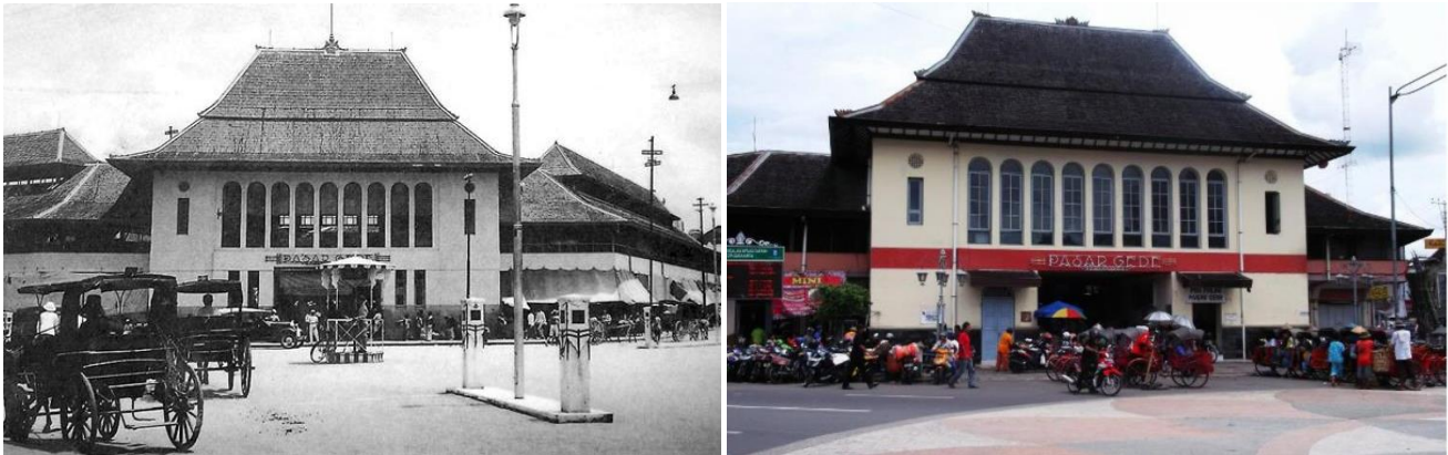
Figure 2. Pasar Gede building, Surakarta, Central Java, Indonesia in 1935 ( left ) and 2022 ( right )
