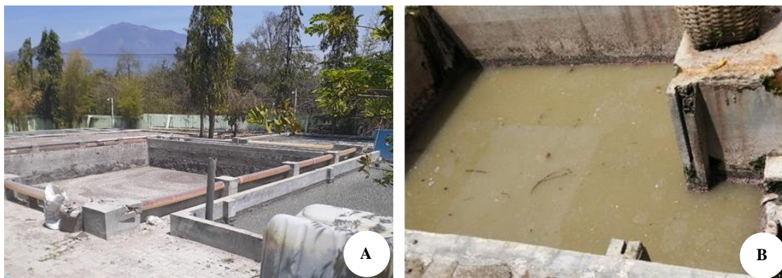
Figure 1. Wastewater treatment plant in a small industrial area in Magetan, East Java, Indonesia. A. Homogenization/equalization tank; B. Homogenization tank wastewater
