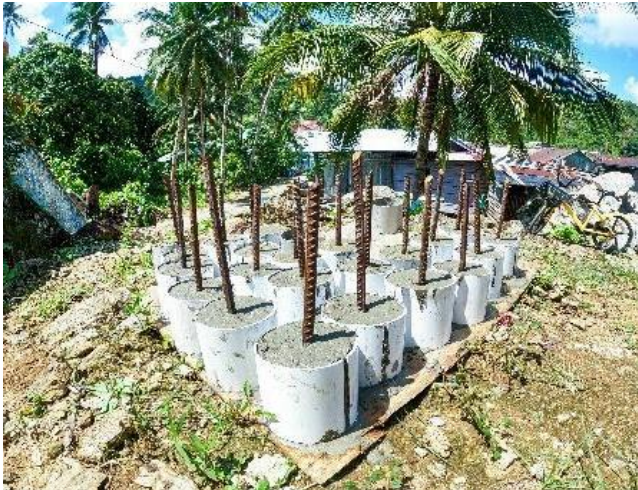
Figure 2. Construction of bored pile coral
