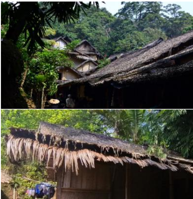
Figure 7. Roof of a Baduy traditional house, Lebak, Banten, Indonesia
