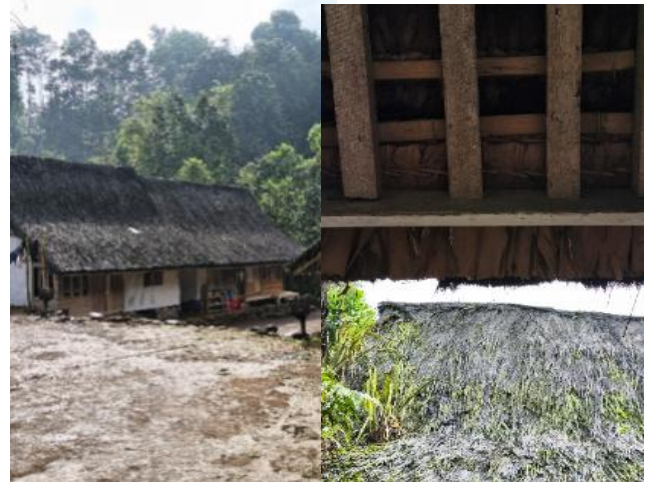
Figure 6. Roof of houses in Kampung Naga, Tasikmalaya District, West Java, Indonesia
