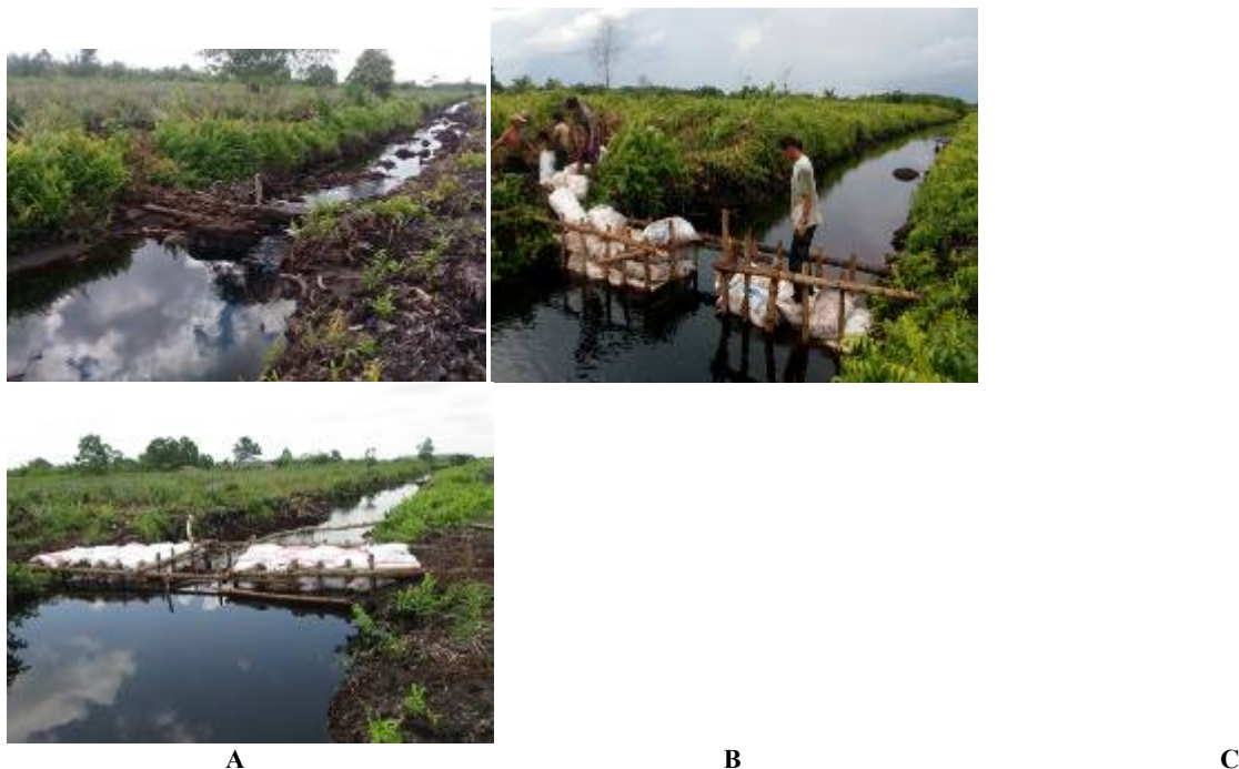
Figure 2. A. A drainage ditch in peatland before, B. During, and C. after the establishment of the water flow-dam
