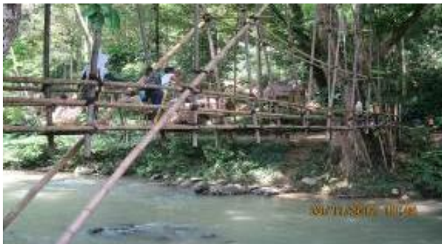
Figure 6. The traditional bamboo bridge of outer Baduy which uses kawung fibers for binding the bamboo
