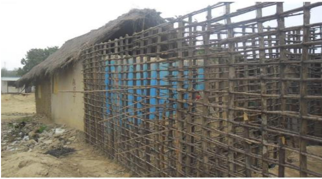
Figure 3. Mangrove trees are used for building at Adakope, Ghana
