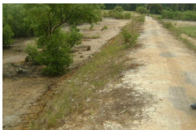
Figure 15. Adaptation strategy of climate change through ridge construction at Ukele, Micheweni District, Pemba Island, Tanzania
