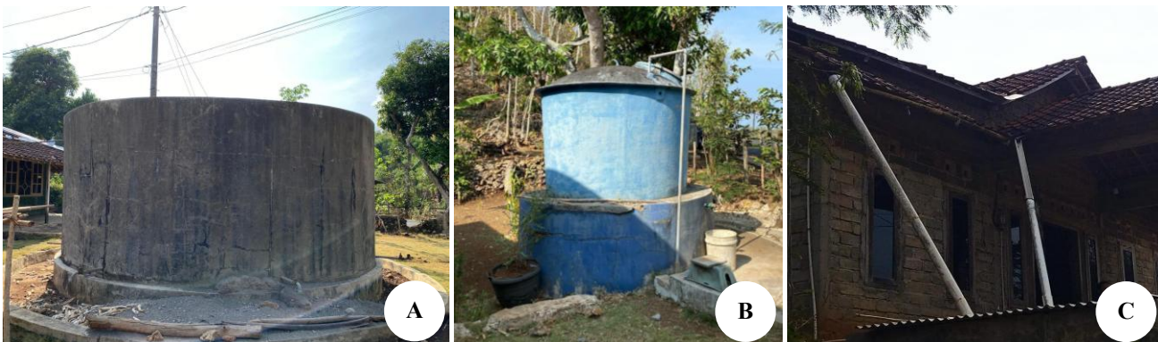
Figure 3. Water management at household level in Paranggupito Sub-district: A. Large-scale water storage tank; B. Small-scale water storage tank; C. Pipes for channeling rainwater into the storage tank
